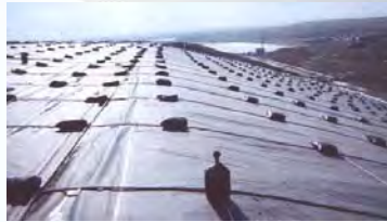
Yolo County landfill near Davis, CA Reinforced Polypropylene Geomembrane
