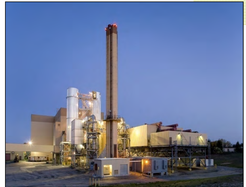
MacArthur Resource Recovery Facility, Islip, NY
