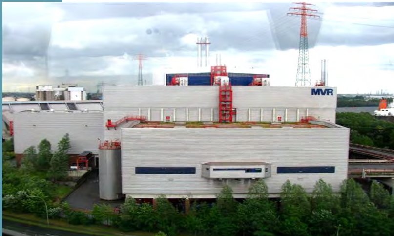
WTE Plant – Hamburg, Germany
