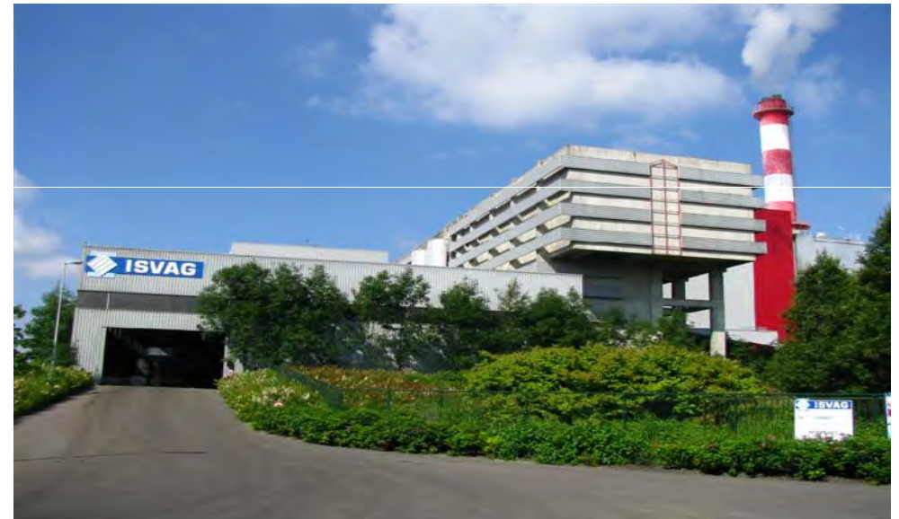
WTE Plant – Antwerp, Belgium
